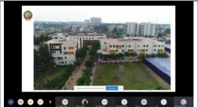
Figure 4: Screen shot of PPT from Speaker explaining the roof top of RRIIT
