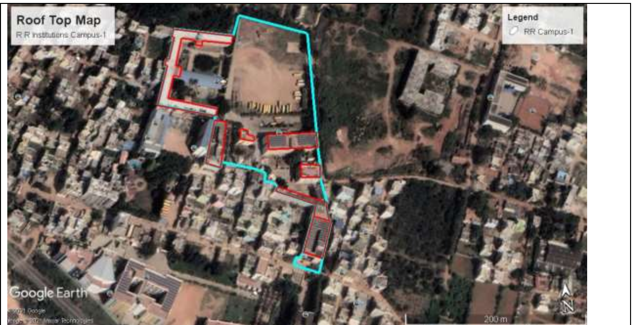
Figure 7: Satellite image of roof top area Campus-1 of RR Institutions
