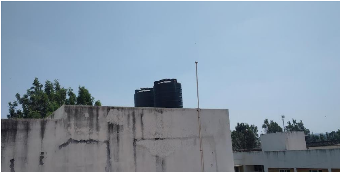
Overhead tank in campus 2
