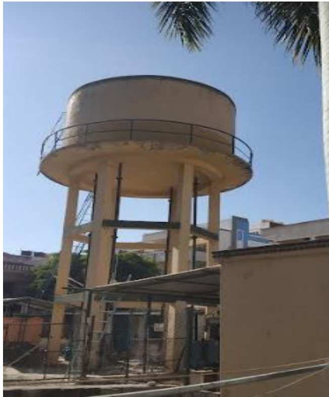
Overhead tank in campus 1
