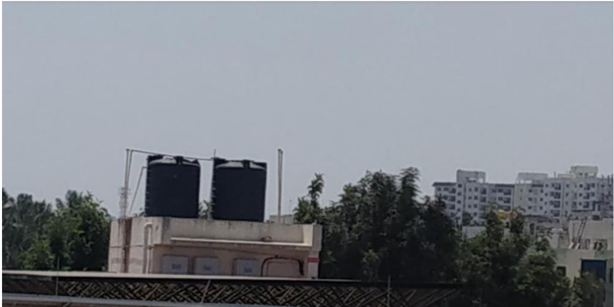
Overhead tank in campus 2
