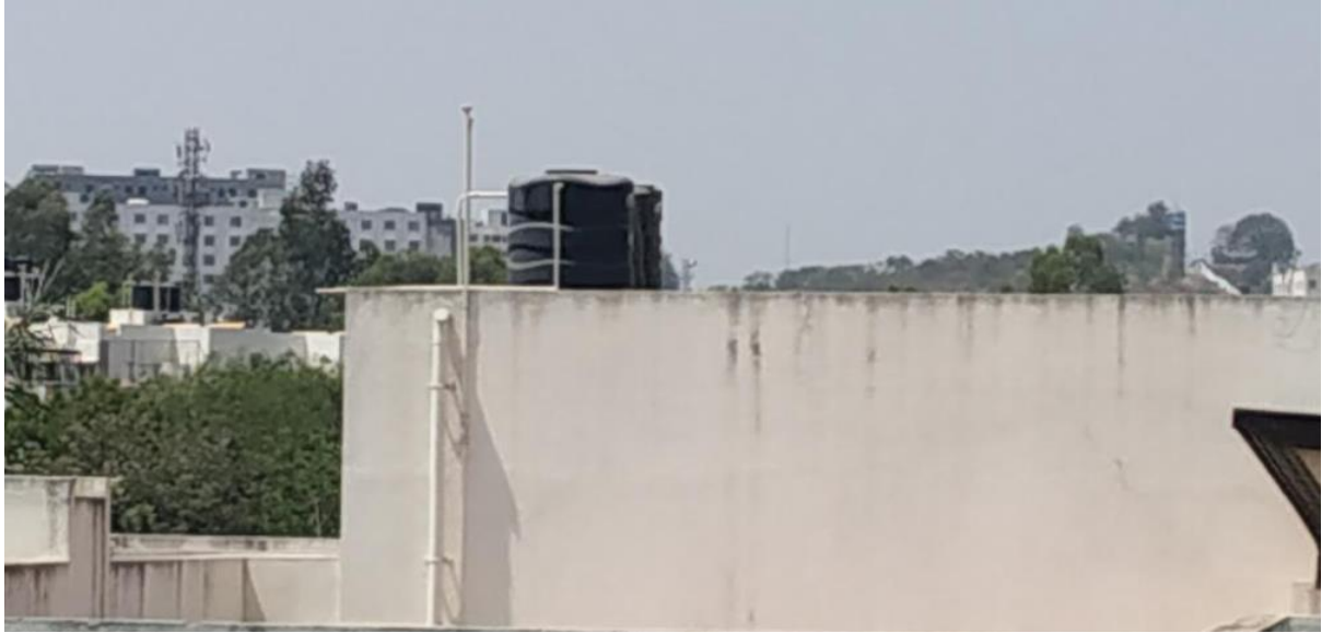
Overhead tank in campus 2
