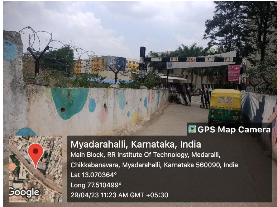
Fig. 2c. College boundary walls
