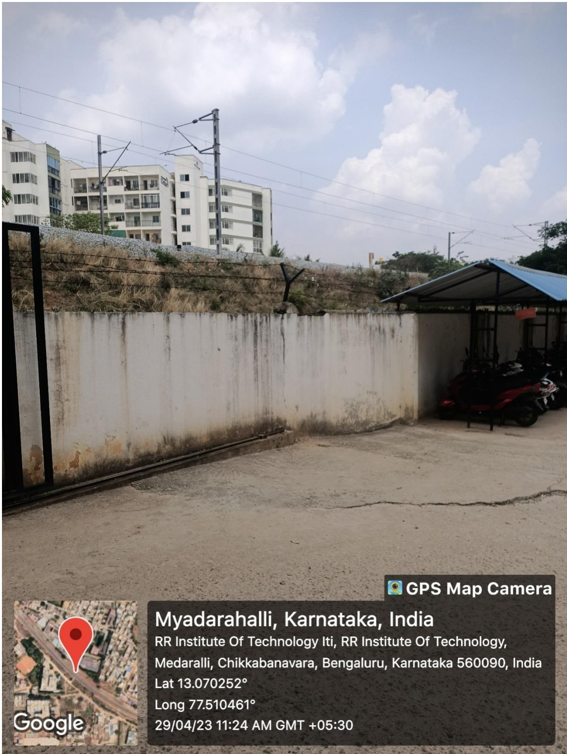
Fig. 2b. College boundary walls
