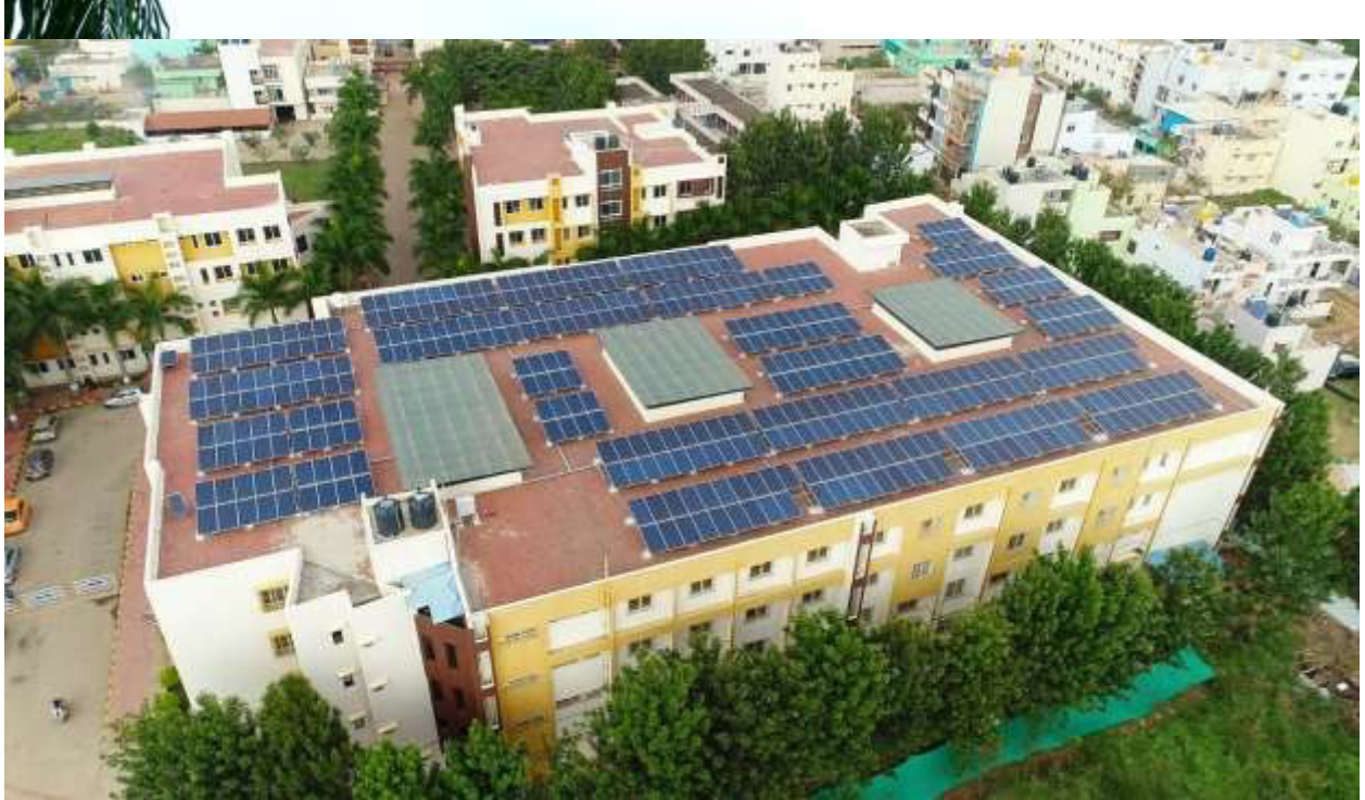
ROOF TOP SOLAR PANEL
